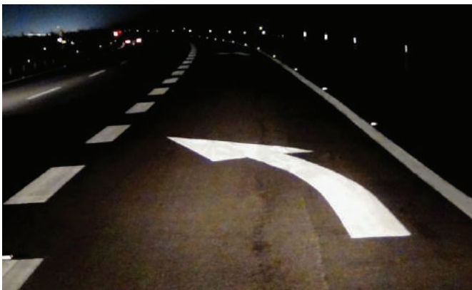
Road marking with glass beads - Nighttime.
