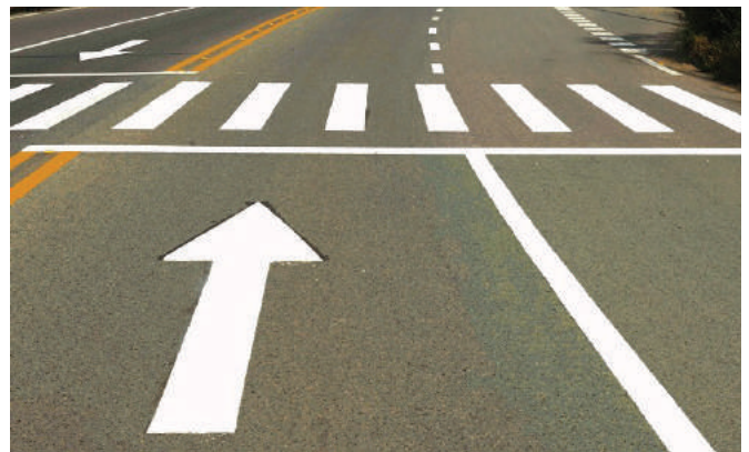
Road marking with glass beads - Daytime.
